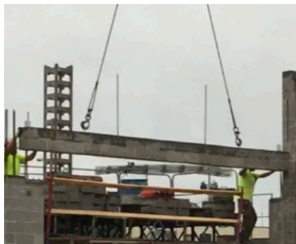
Figure 1: Prefabricated Masonry Lintel
