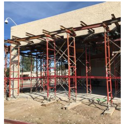
Figure 1: Needle Shoring at New Masonry Opening
